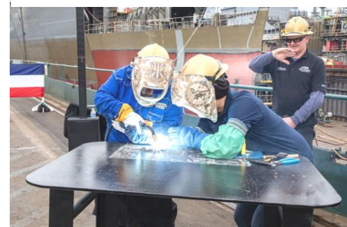
Initial Welding on Steel Plate.
